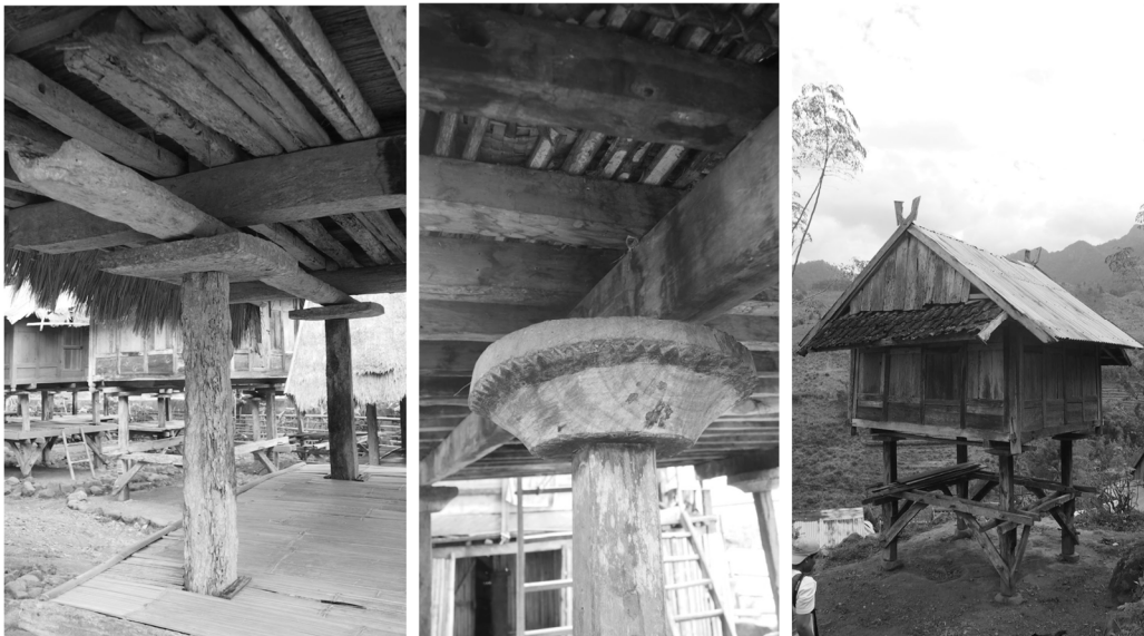
Figure7: The micro arrangement as a response to food making--the Ri'i wooden pedestal and the arrangement of the wooden ladder Source: Author
