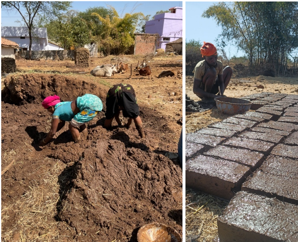
Figure 5: As shown in the picture above, the process of preparing mud bricks is being demonstrated.
