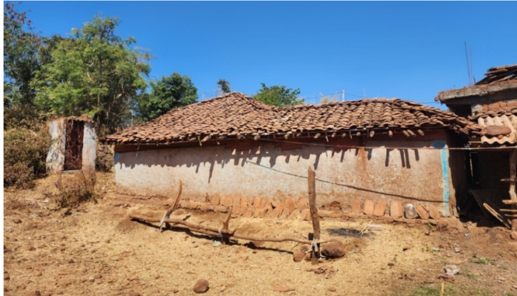
Figure 1: Vernacular Architecture house built with organic, inorganic, and composite materials.
