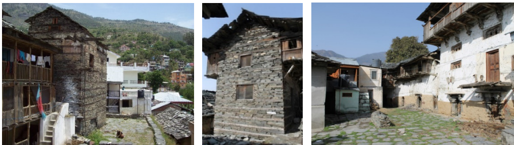
Figure 11: Built forms with Stone and Timber Construction, Village Nirmand
