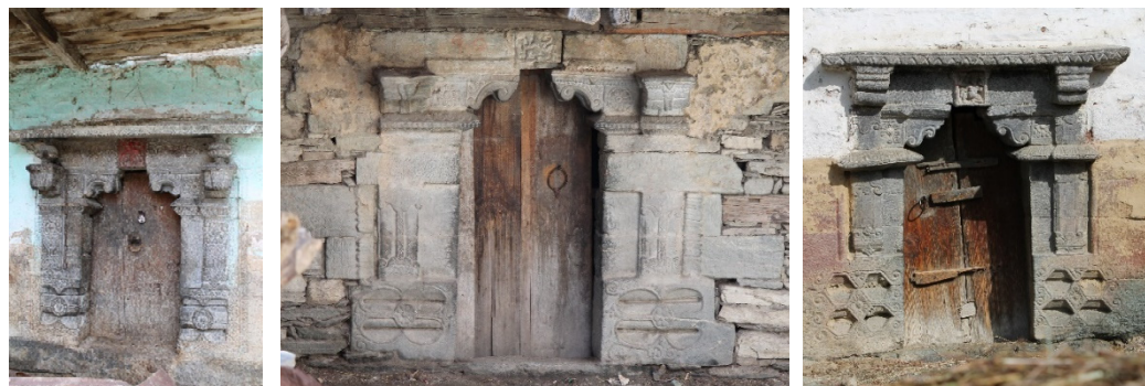
Figure6: Traditional Entrance Doors with Small Size, Village Nirmand
