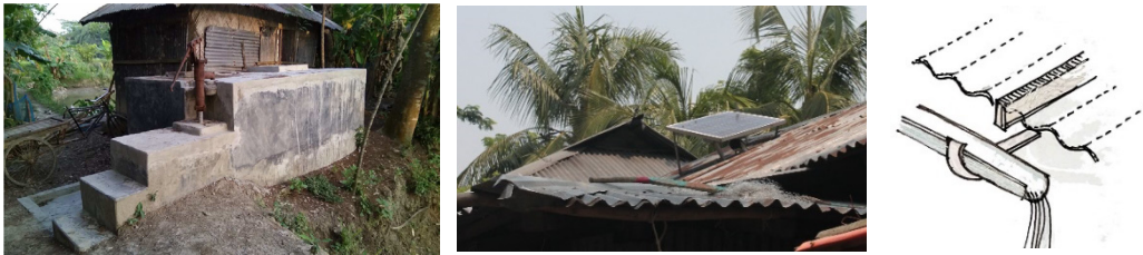
Figure 8: Traditional techniques of rain water harvesting, protecting roof from wind and use of solar panel.
