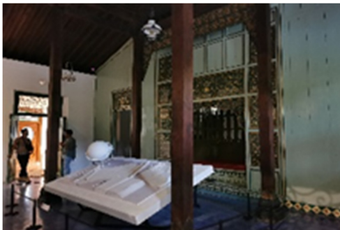
Figure 4: The Joglo surrounded by masonry walls.
