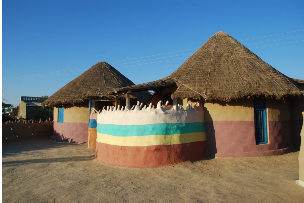
Figure 1: Vernacular Architecture built by Bhogha Tribe, made of mud, husk, grass and twigs Photography by Mr. Ashish Patil, Bhogha Tribe, Rajasthan India
