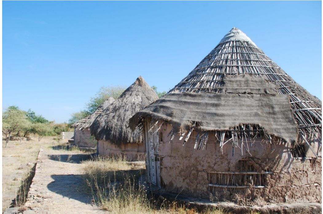
Figure 3: Vernacular Architecture built by Bhogha Tribe showing the skin of the hutment. Source: Mr. Ashish Patil, Bhogha Tribe, Rajasthan India
