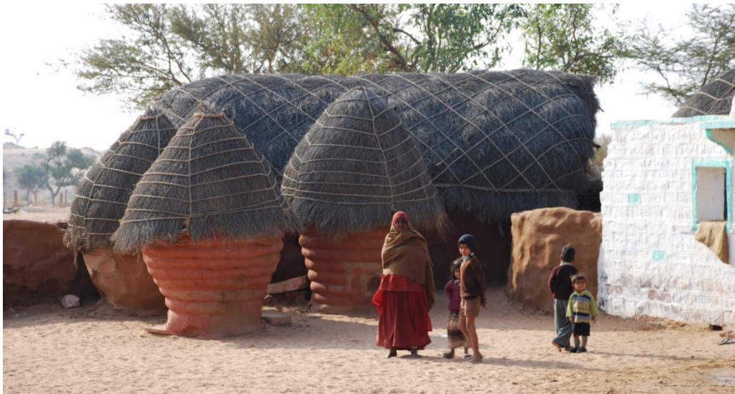
Figure 2: Vernacular Architecture built by Bhogha Tribe, made of mud, husk, grass and twigs (another view)
