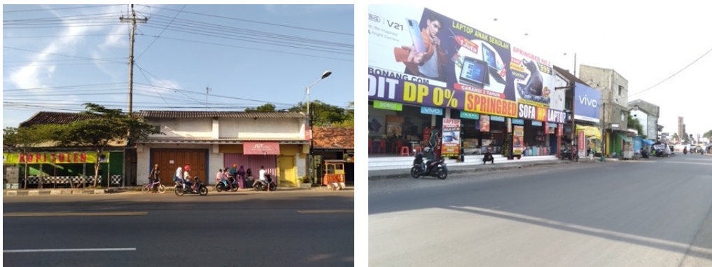
Figure 3: Shophouse buildings along Jalan Pantura and Jatirogo Lasem Source: Author
