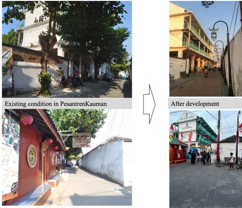
Figure 13: The loss of shade trees in the area of Pesantren Kauman, Lasem due to physical development. Source: Author
