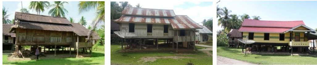
Figure 17: Godang House Renovation Process from time to time in Koto Sentajo Source: Faisal, et al, 2018
