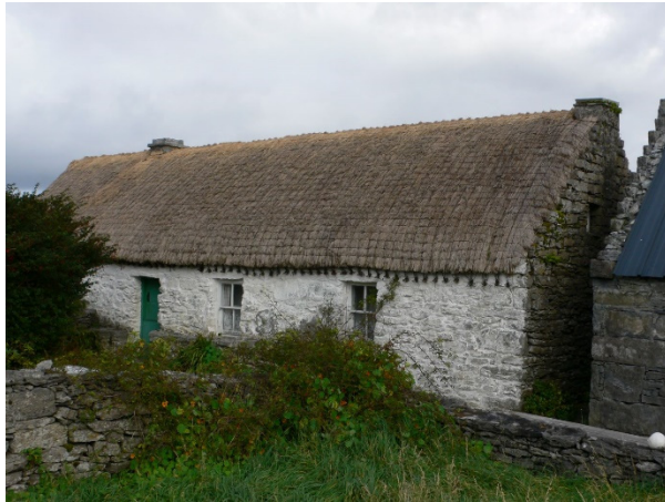
Figure 1: Roped thatch house, Aran Islands, County Galway Source: National Inventory of Architectural Heritage
