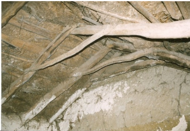
Figure 3: Typical historic roof of rough boughs, set into wall tops, near Tullamore, County Offaly
