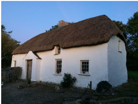
Figure 2: Thatched house with thrust thatch roof, Mayglass, County Wexford Source: Barry O'Reilly
