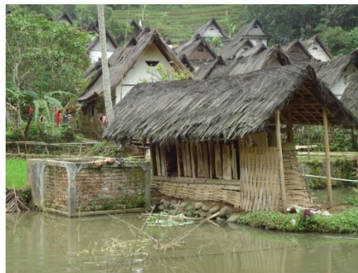
Figure 6: Outside kandang jaga (dirty, watery) Source: Saraswati's Documentation
