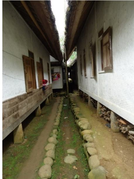
Figure 16: Narrow hallway behind houses
